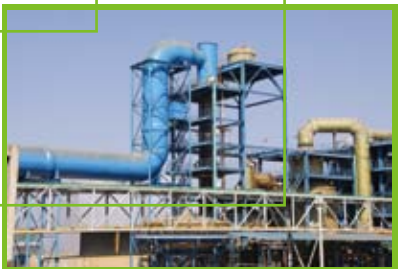
Sulfuric acid absorption tower
