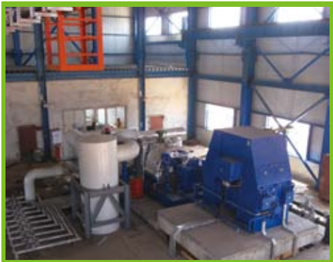
A waste-heat power station --- providing approximately 18% of the electricity consumed in the plant area
