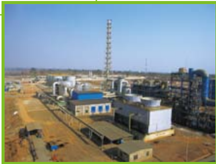
All fumes from copper smelting are used to make acid
